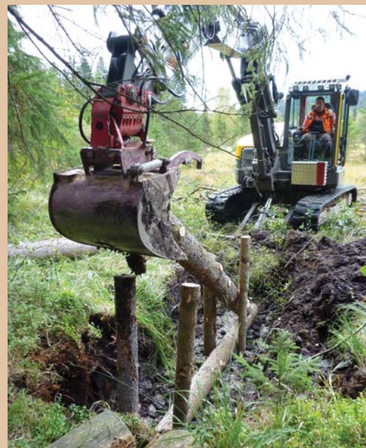
Construction of a log dam
